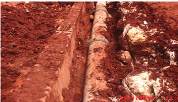
Water & Electrical Installation
