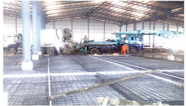
Ground Floor Concrete
