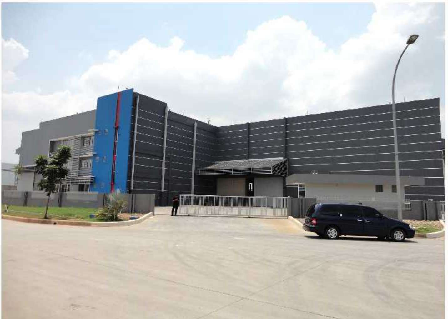
Warehouse - PT Hextar Fertilizer, Cikarang LT: \pm 12.500 \text{ m}^2 LB: \pm 10.000 \text{ m}^2
