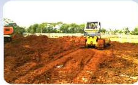
Cut and Fill
